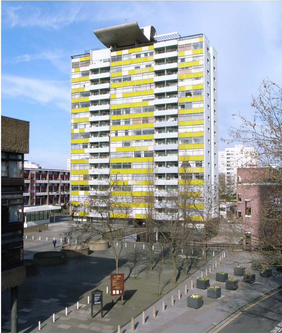
View from the north of Great Arthur House
