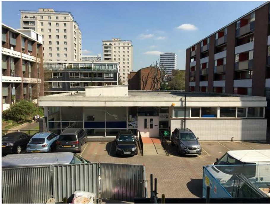
Front elevation of the Community Centre
