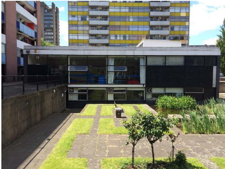
Rear elevation of the Community Centre
