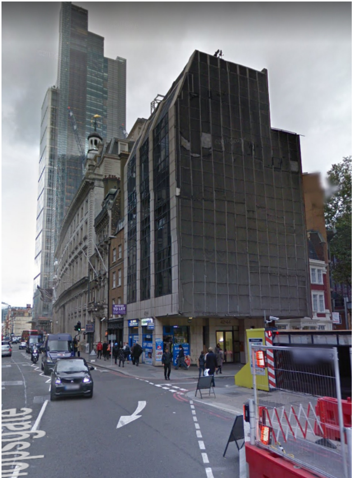
Appendix 2 –Image; Flank Wall 42-44 Bishopsgate, EC2
